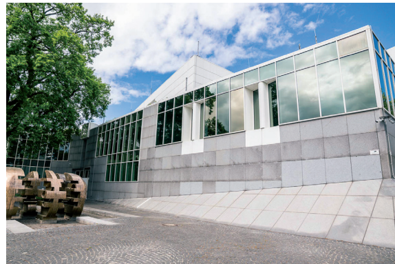
The VIVAVIS data centre is located in the former vault of the Hessian regional bank.
